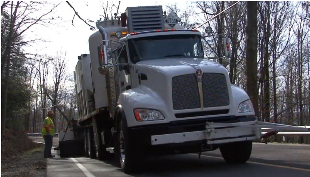
Figure 5: Application of an HFST by truck.
