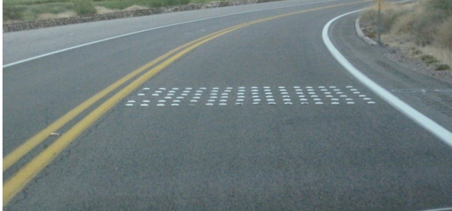
Figure 78. Photo. Additional traffic calming installed between 12 and 24 months at SR 95.
