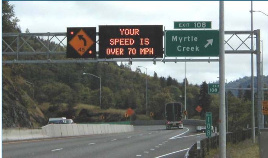
Figure 28. Photo. Interstate 5 DSFS systems in Oregon (Northbound after).
